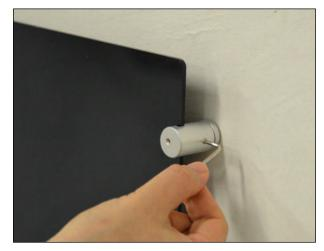
**4.** Finally, tighten both grub screws on each of the upper stand-offs to fasten the sign in place
