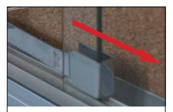
**3.** Slide the top door over the notched bar. Slide both doors until the end.
