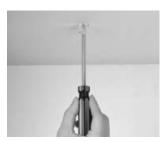
Determine the position of the sign and drill a hole for each fitting into the ceiling. Screw the top half of the fitting into the ceiling.
