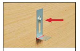
Remove the noticeboard. Align the L-Bracket with the marked position. Screw the L-Bracket into the wall.
