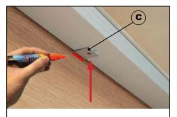
**5.** Align L-Bracket to the holes underneath the noticeboard and mark the position on the wall.
