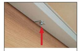
7. Mount the board on the wall and screw the L-Bracket to the board to secure the board on the wall.
