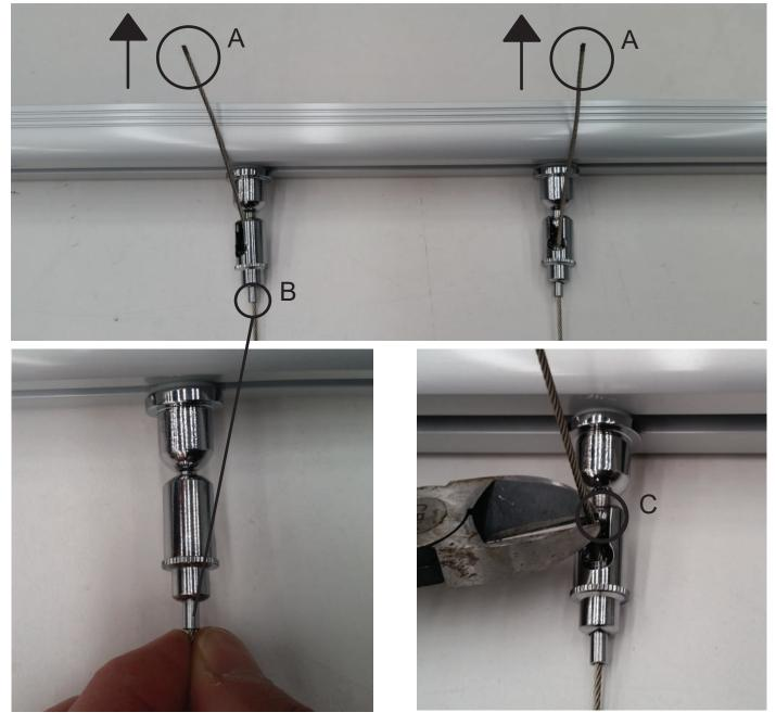
4. Adjust Lighboxes to desired height by pulling cables upward (A), to shorten cable depress part (B) 5. Once desired height is achieved and installation is complete, trim Top cables inside knuckle C.
